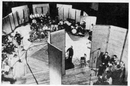
ACOUSTIC SCREENS are set up in the studio to control reverberation and separate the chorus in the foreground from the orchestra in the rear. The conductor is stationed centrally, visible to all musicians,
