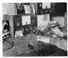
FIG. 8: Reconnect the wire leads to the motor coil soldering terminals and replace the unit into the radio.
