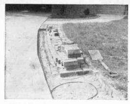
FIG. 7: Brick walk alongside driveway helps simplify problem of bedding down the pickup coil and cable.
