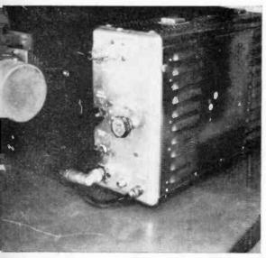
Fig. 4: A surplus selsyn is used to focus the camera lens remotely. Useful if camera is out of arms reoch.
